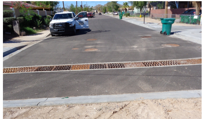
Completion of South Calle Sahuaro
